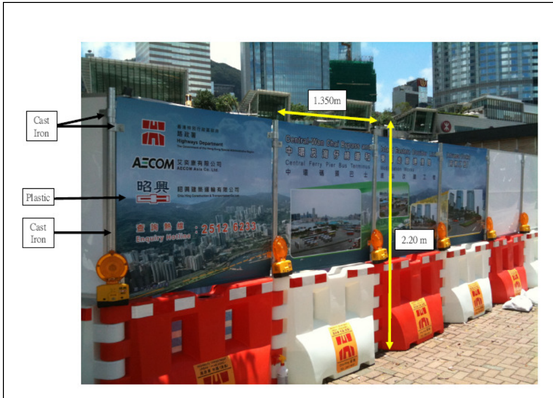
Design and dimensions of the Decorative Screen Hoarding
